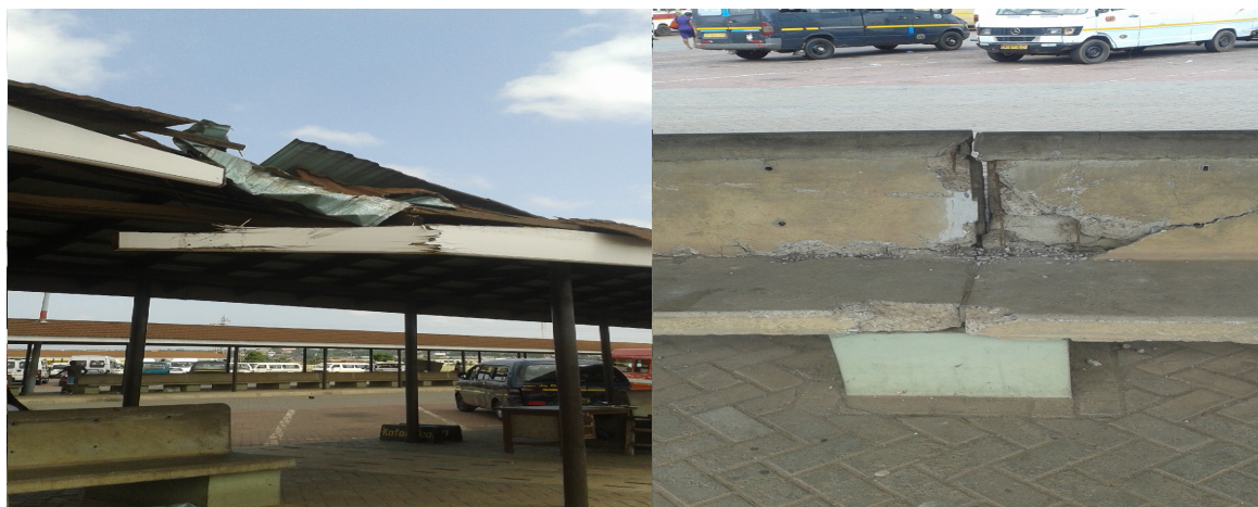
Figure 3. Showing the defect to the roof and concrete bench
