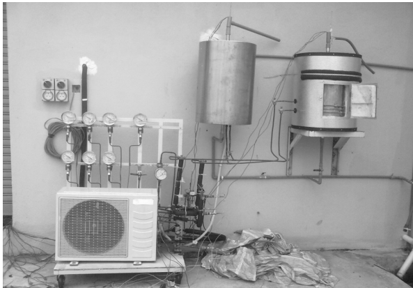
Figure 2. Photograph of condensing outdoor units
