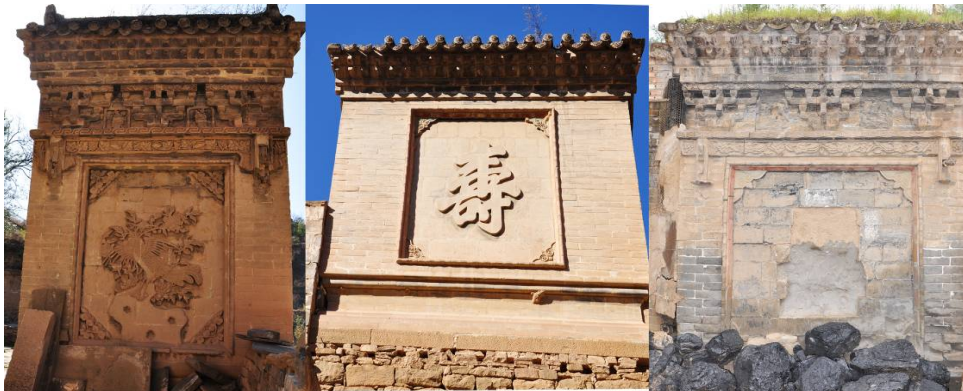
Figure 3. Tile carving of the screen wall in Dangshi manor (source: drawn by the authors)
