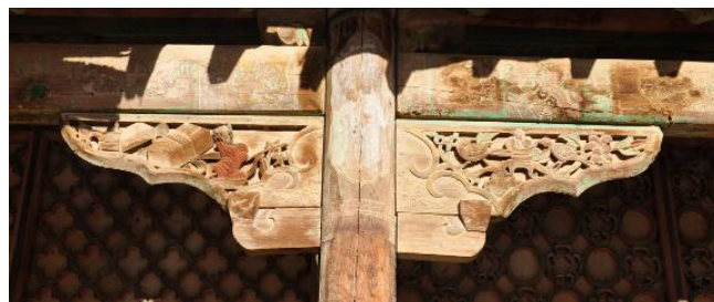
Figure 6. Wood carving of the sparrow brace in the wing-room of the major courtyard (source: drawn by the authors)
