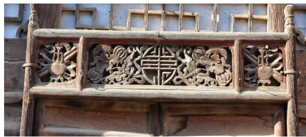
Figure 5. Wood carving of the lintel in the front cave dwelling of the major courtyard (source: drawn by the authors)
